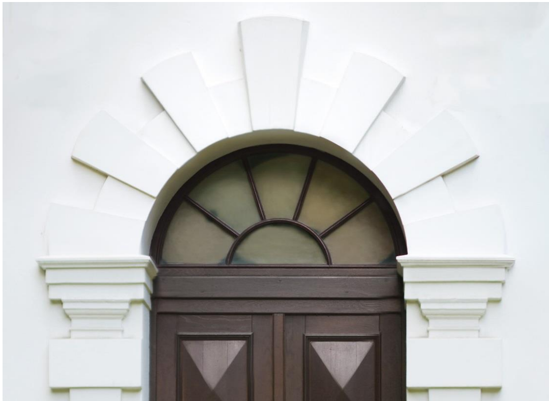
Figure 23: The installation of the perceived greys in the arch window.
