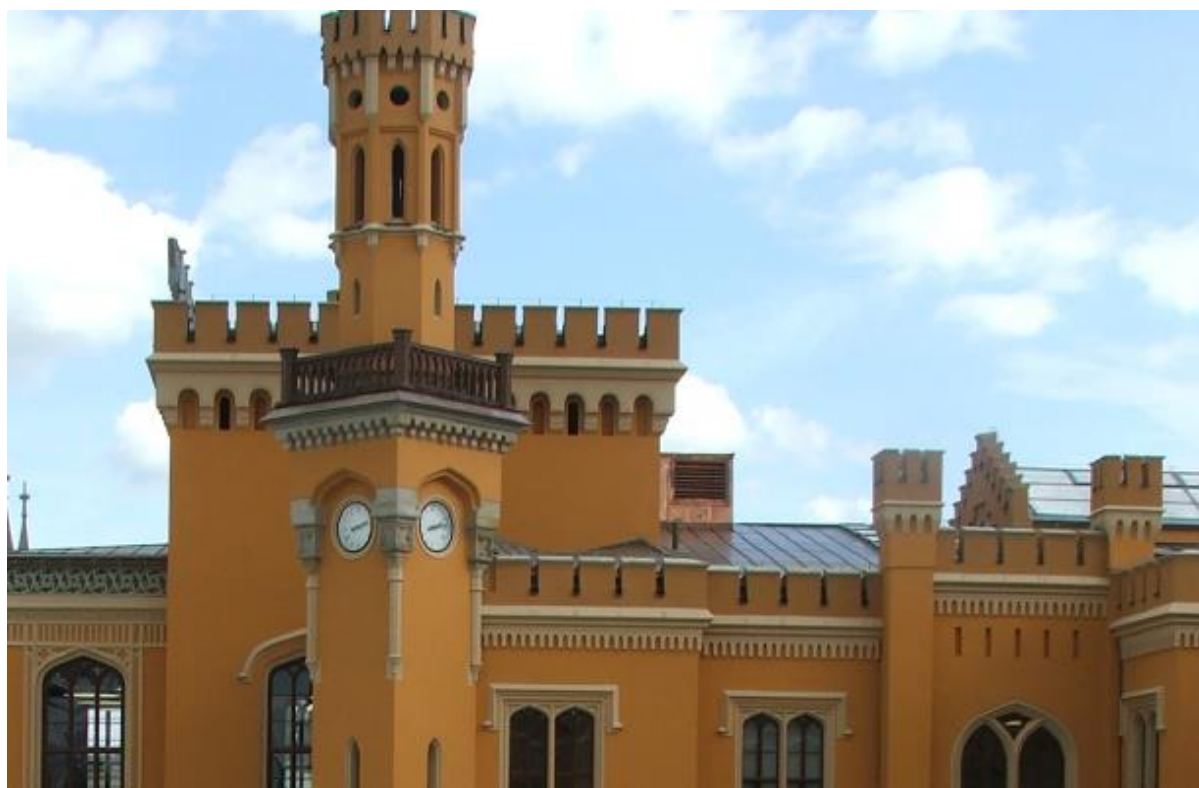
Figure 8: The railway station Wrocław Główny - detail. The elevations were partially restored to the original colour scheme from the mid-19th century. The colour scheme was possible to detect due to the full access to the building.
