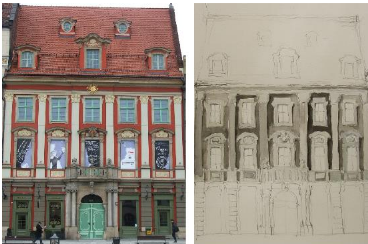
Figure 10: 6 Rynek, Wrocław. The building has been rebuilt and redecorated a few times since the Middle Ages. The second examinations revealed traces of colour schemes: red-pink paint (1st phase) and light yellow ochre (2nd phase), both possibly from the period before the Baroque refurbishment. The dark grey and grey colour scheme was discovered directly on the Baroque window surrounds (Photo and sketch by the author, 2013).
