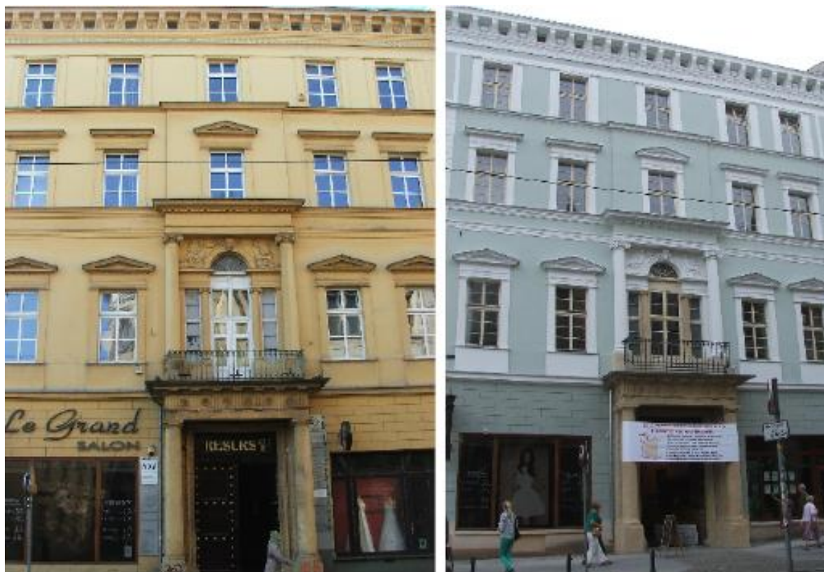
Figure 7: 16 ulica Wita Stwosza, Wrocław. Yellow ochre was estimated as the original colour by on-site observations (left). Re-examinations with the analysis of selected samples under the microscope revealed that the building was originally painted monochromatically grey-green. The grey-green layer of paint was visible beneath yellow ochre under the microscope (Photos by the author in 2012, 2015).
