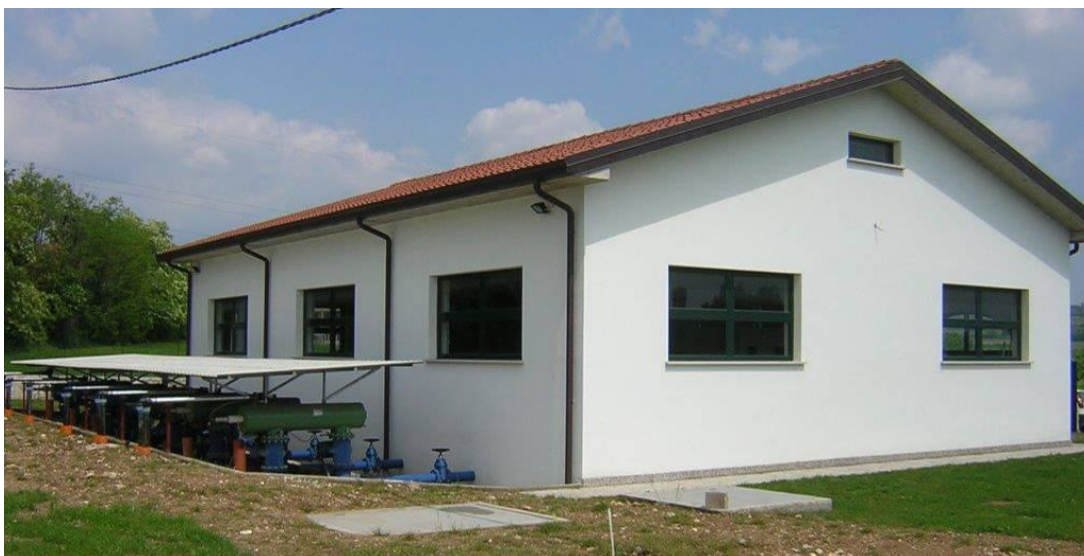
Fig. 5 – Small pumping stations contemporary building, Castelnuovo del Garda, VR (photo © A.Piva)
