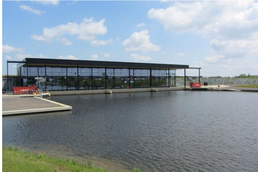
Fig.8 –St German pumping station, London (photo © A.Piva)
