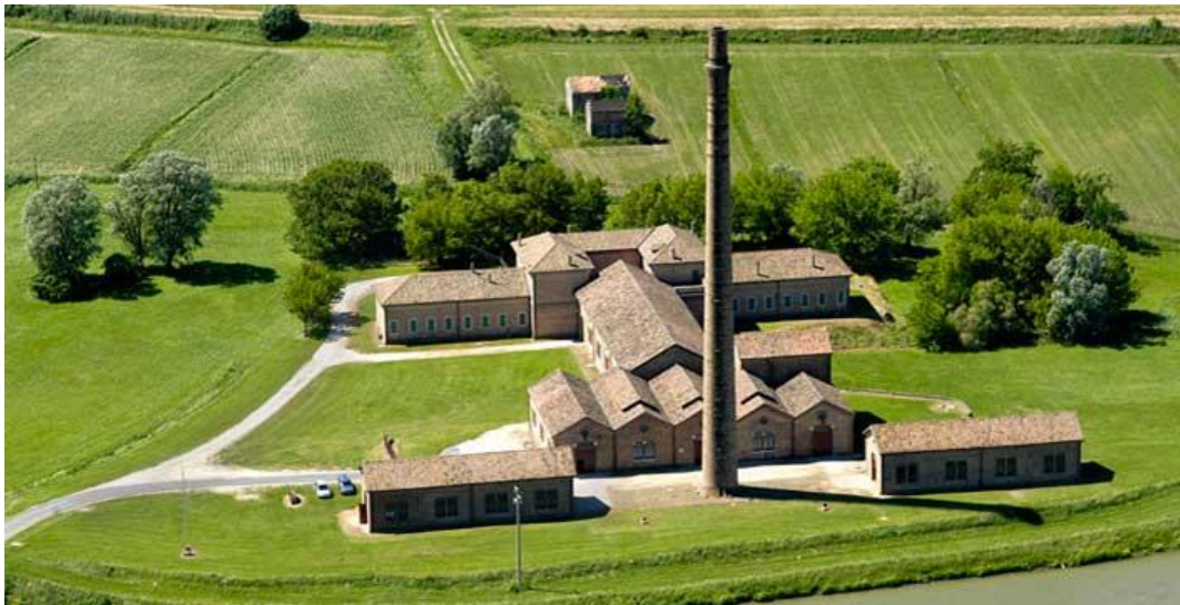
Fig. 3 – Cà Vendramin pumping station, 1900-1905, now houses of the Reclamation Regional Museum (photo www.fondazionecavendramin.it )
