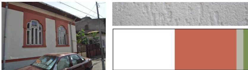
Figure 7. Photographic survey of the colours and textures and of their proportions 22 Bahluiului street
