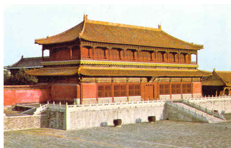
Figure 2: The Hong Yige building in the Forbidden City. Photo by Maria do Céu Rodrigues.
