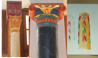
Figure 1: Columns' capitals after reconstruction. Photo by Dorota Kozak. Column shaft detail- Reconstruction of original colour schemes by author based on results from examinations.
