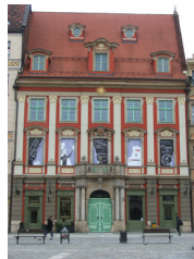
Figure 2: Wroclaw, Rynek 6, front elevation. During lasted refurbishment colour scheme did not follow the examination results. Photo by author.
