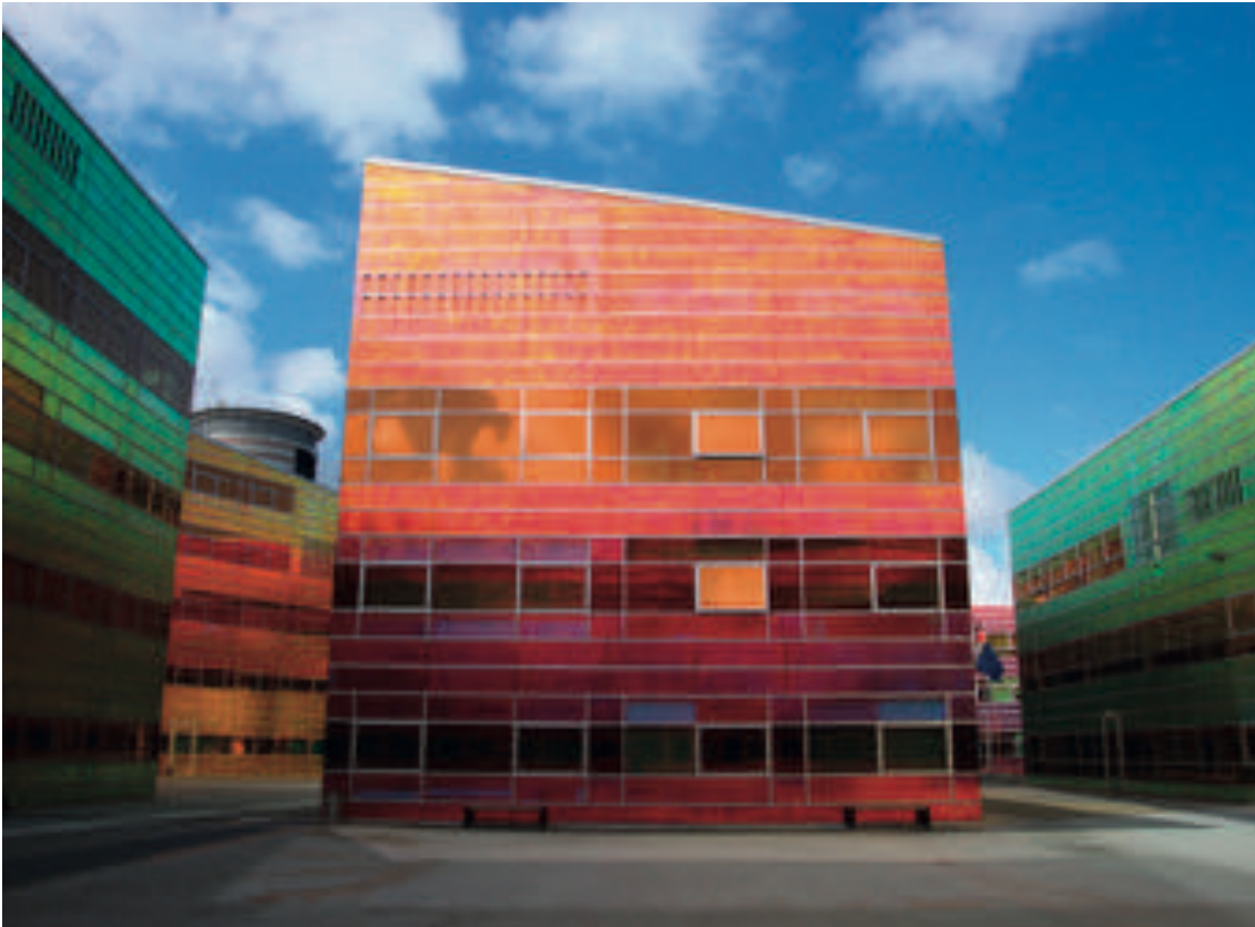
UN Studio, La Defense Offices in Almere, Netherlands (2004) Photo: Author
