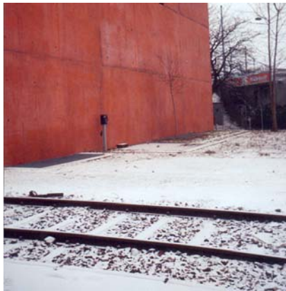
Fig. 7 Wall of iron oxide coloured concrete.
