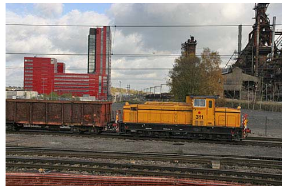
Figure 3 The bank center of DEXIA by Vasconi on an old iron and steel pole of Belval in Luxembourg.
