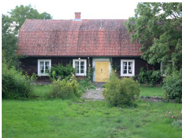
Figure 3. This dwelling is from the beginning of the 19 th century, with the wooden construction visible and tared. Together with the white windows and polychrome main entrance, it is a typical local colouring at Öland during the period.
