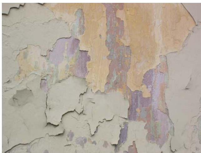
Figure 2. This detail of a plastered facade, from a farmer's house in the coastal region of southern Sweden, shows many of the old layers of paint in many different colours.
