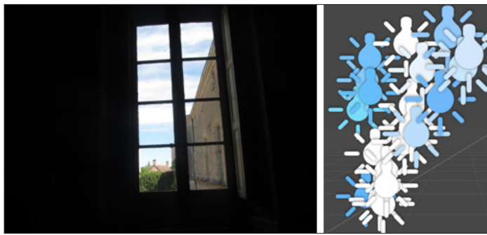
Figure 2: An image of the window of the north wall (a) and point source sampling (b). The colour of the point light sources reflects the dominant blue colour of the window.
