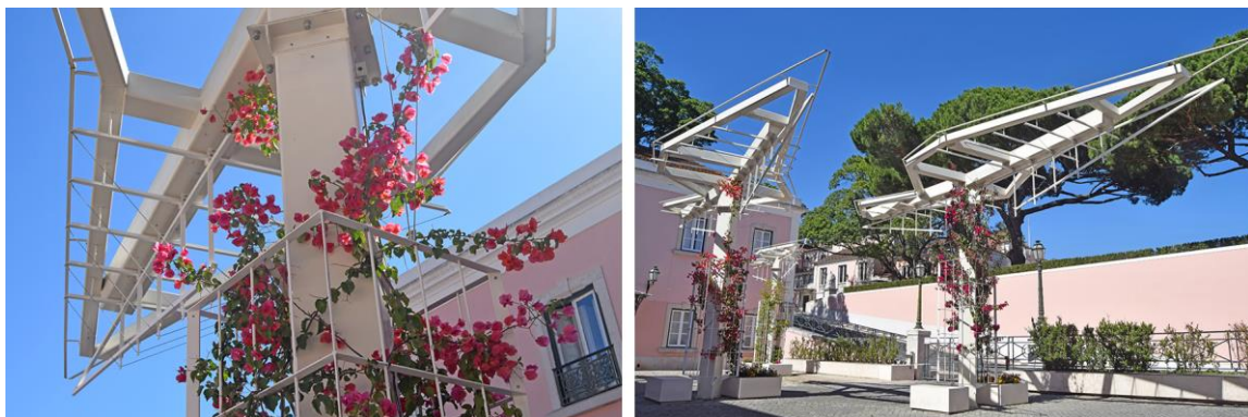
Figure 5: Museum of the Presidency of the Republic, Lisbon. Rehabilitation of the metallic trees: evolution of the bougainvillea growing. Photos by R. Barreiros Duarte, 2019.
