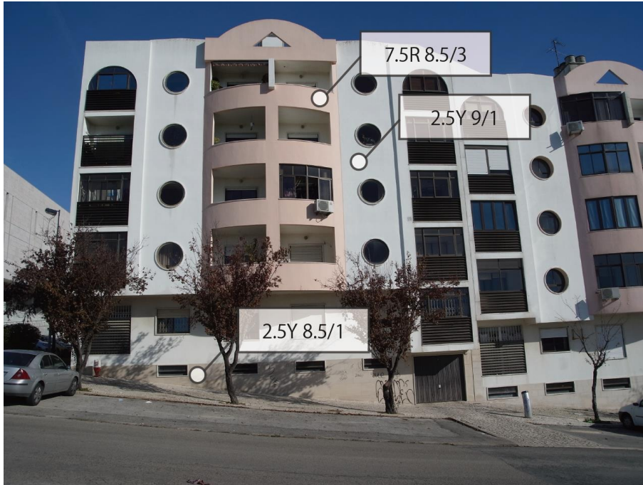
Figure 1: An example of surface color measurement results of an apartment building in the color survey.
