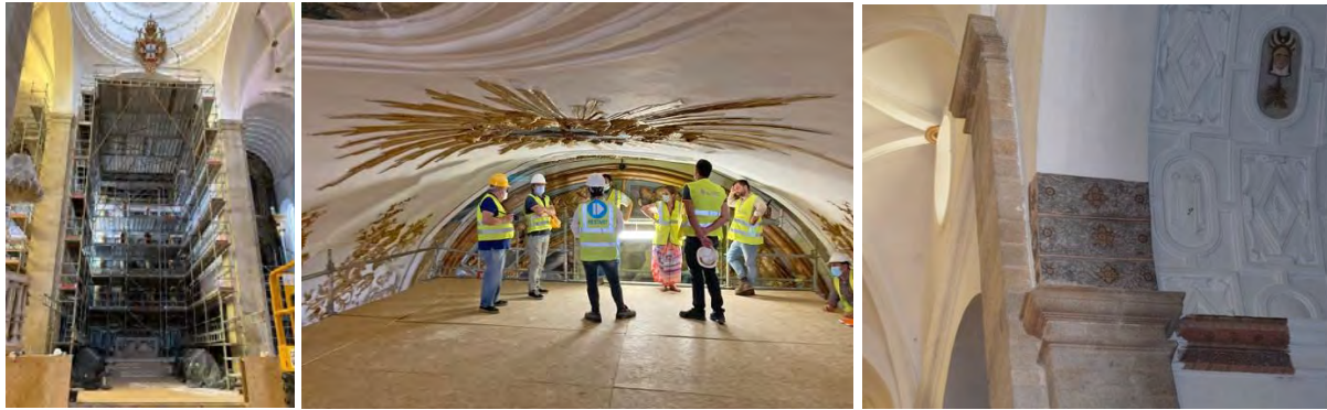
Figure 5. Chancel (left). Chancel vault (center). North chapels (right). Photo: RBD.APP, 2022.
