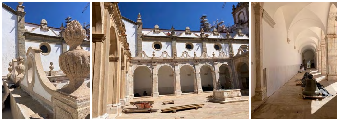
Figure 4. Rooftop (left). Cloister (center). North gallery of the cloister (right). Photo: RBD.APP, 2022.
