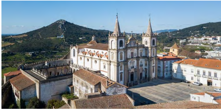
Figure 1. Rehabilitation of the Cathedral of Portalegre, its cloister and annex spaces: 1 st prize in a competition by invitation. Architects: RBD.APP, 2014. Photo: João Morgado, 2020.
