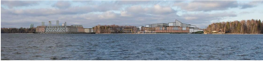
Figure 2: The cityscape with SkechUp-model with the previous picture. On the left side of buildings will be four white skyscrapers at Keilaniemi in Espoo.
