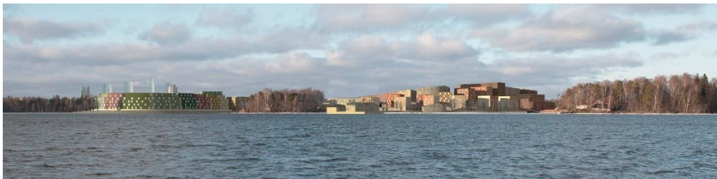
Figure 3: The right side with yellow-red-brown-scale has remained the same in the last version. The left side with green buildings has developed in the next steps of planning. The detailed plan is going to City Board in 2019, so unfortunately the pictures of the next four steps are not public yet.
