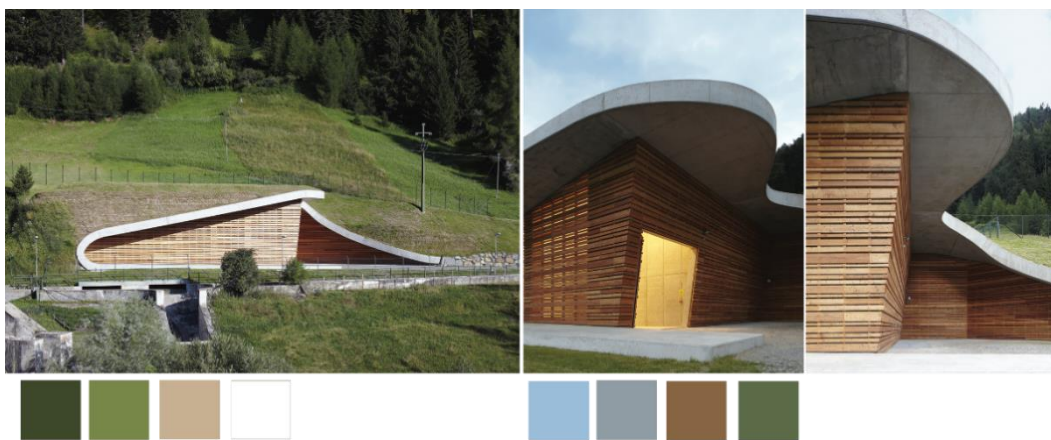
Figure 1: Punibach hydroelectric power station (ph.© MONOVOLUME Architecture+Design).
