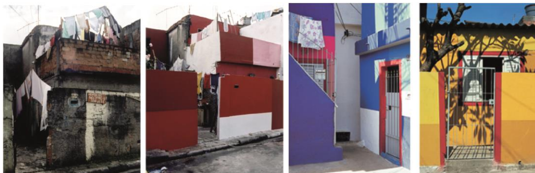
Figure 1: Façades of the favela of Heliópolis before the painting and the final result after the colours application. Source: Ruy Ohtake (2012).
