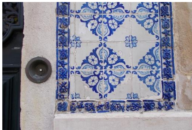
Figure 1: Rua da Imprensa Nacional 96, detail of the glazed tiles.
