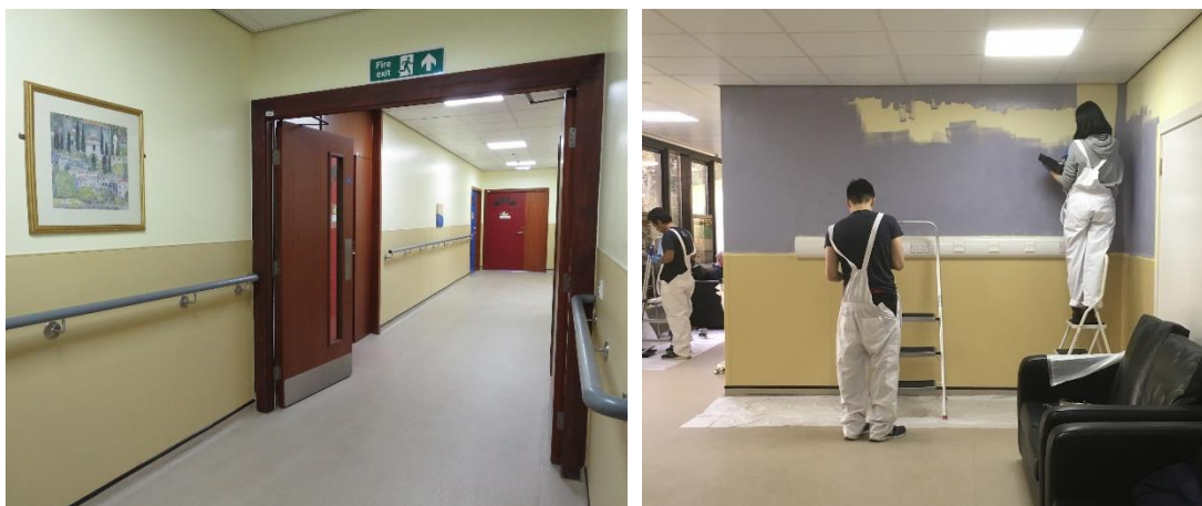
Figures 1 and 2: Circulation before installation, students painting.
