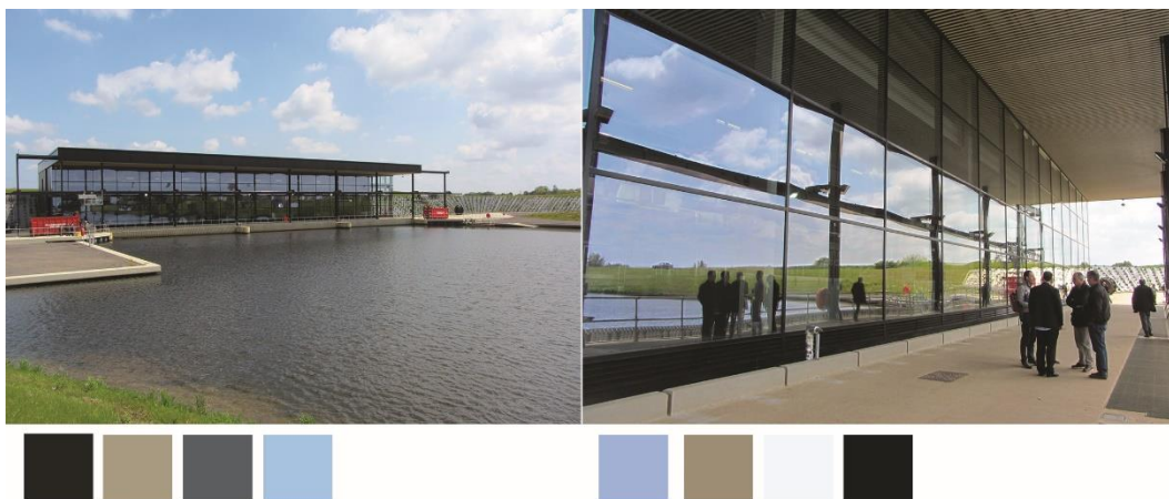
Figure 4: St. German Pumping Station, environmental colour reflection (ph.© A.Piva).
