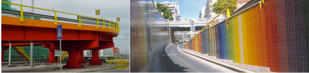
Figure 16. Structure and detail from Eduardo Nery tiles' viaduct mural
